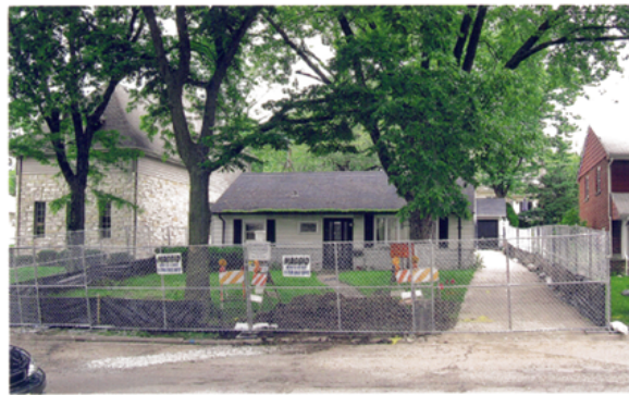
BEFORE The old one-story house at 619 South Bruner Street in Hinsdale before it was demolished.
