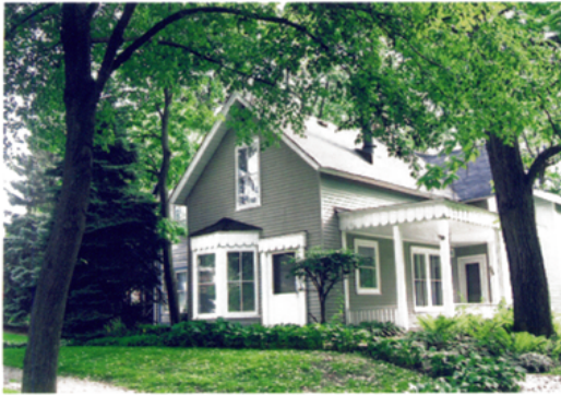
BEFORE The old house at 444 South Adams Street in Hinsdale, Ill., a village 20 miles west of Chicago.
